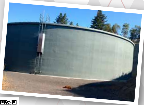
Prestressed Concrete Storage Tanks
