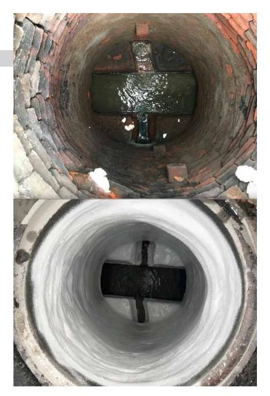
Every time we go out to rehab a structure, whether that is a manhole, lift station or just a chunk of concrete missing from a wall. We get to take something that was damaged or failing and with the help of some great products, not only turn that into something usable again, but also give that structure a much longer life. •
