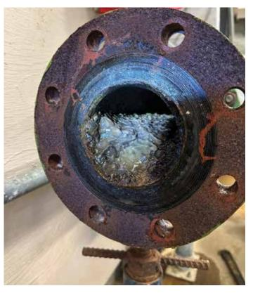
reinstalling it. After unbolting and removing it we will be able to see if it is caked up. If it is stainless steel and has heavy deposits, a flat head screwdriver may be useful, but if it is fiberglass or plastic you may want to be more careful during this part.
