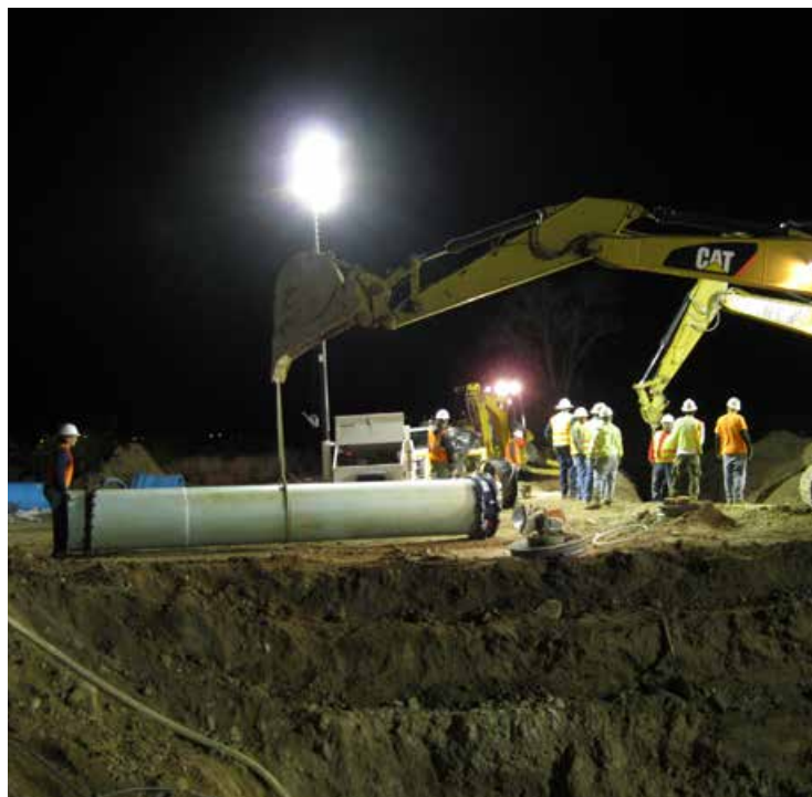
Use floodlights to illuminate areas where crew will be working.
